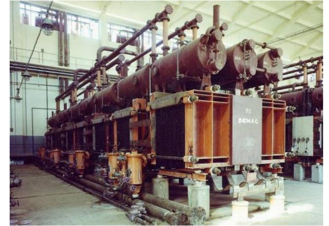
› Demag-elektrolyser @ Aswandam Egypt, 1959 largest electrolyser ever build 203 MW .(Photo Thijs de Groot)
